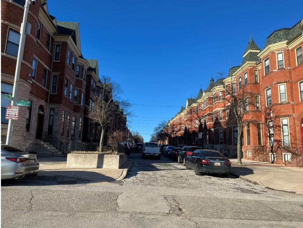
Figure 11: Rowhouses along Callow Avenue, view looking north.
